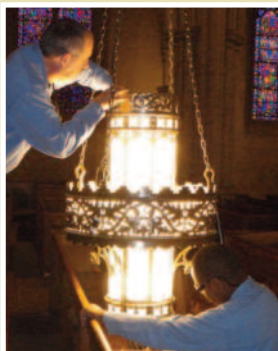
Tom Huff and Abiathar Wade test bulbs before Ron Hurdle cranks the chandelier back into place.
